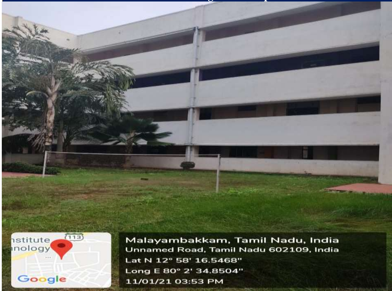
Rain water harvesting collection points
