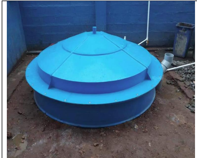
Biogas plant – 100 kg capacity
