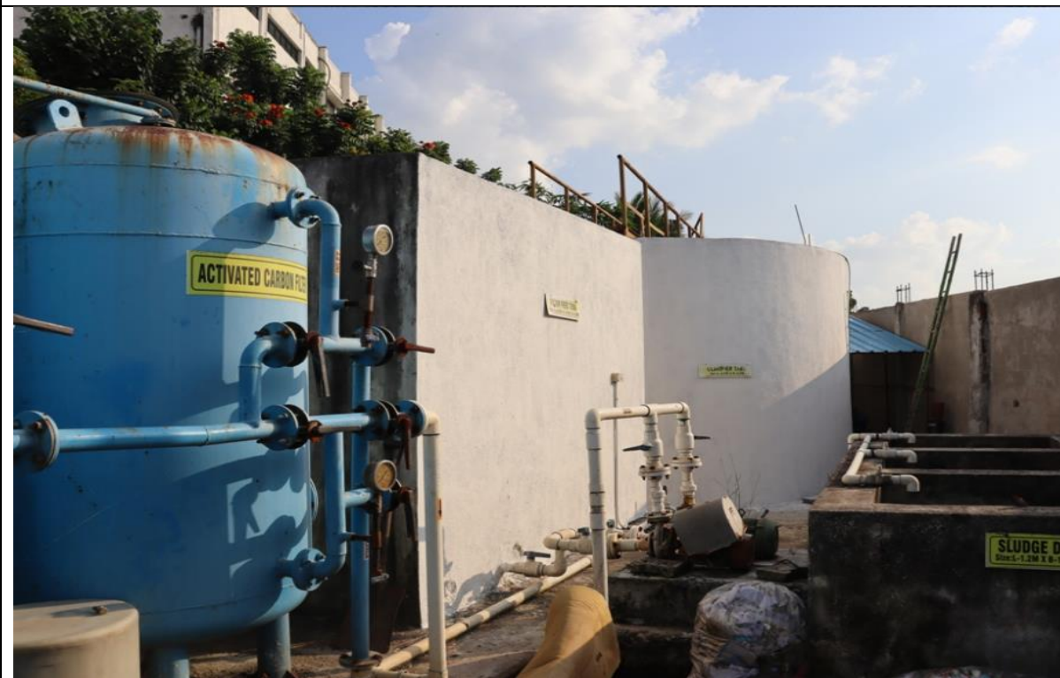
Pressure Filter Units
